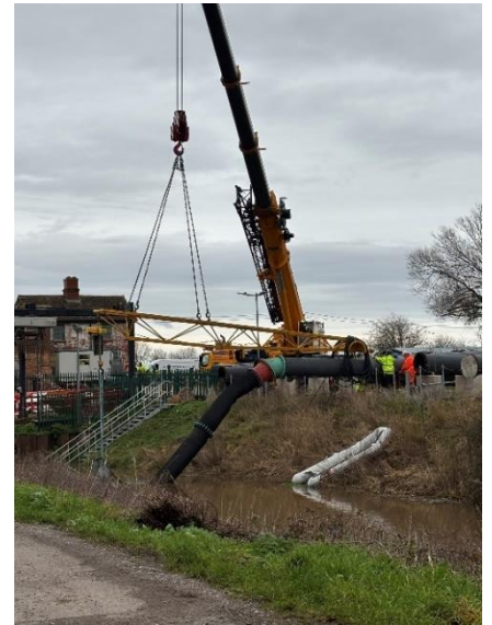
Crane in operation at Northmoor today (Monday 26 Jan)
